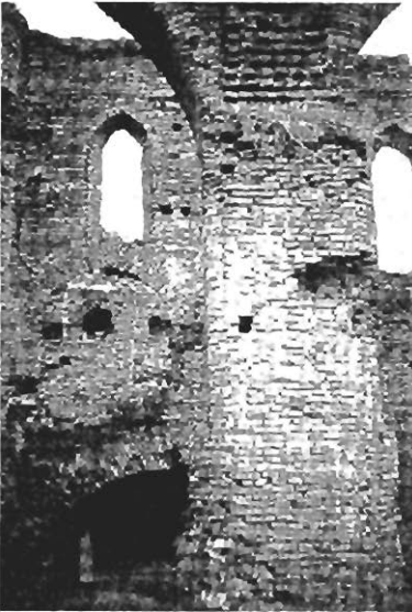
Fig. 2. The eastern side of the northern tower. The Gothic arch is bricked up and a basement room has been created inside the wall itself.
