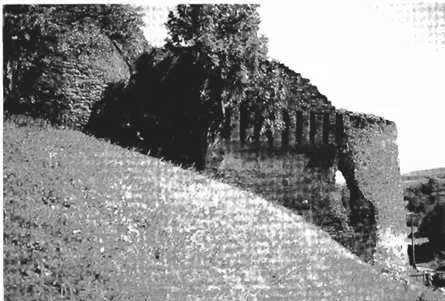
Fig. 4. The southern tower and the buttress that separates two periods of construction.
