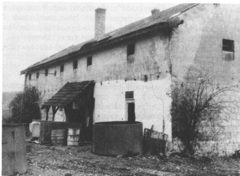
Fig. 3. Boiler of a CO-OP. Tyukod (Szabolcs County) Photo by Géza Balázs
