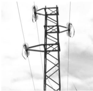
Type 1. Metal structure with jumper wires and 3 lines
