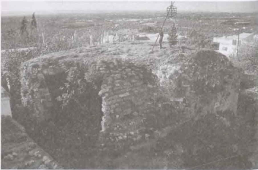
1. Burġ Mi'ār Šakir – ground floor of the tower from the southeast
