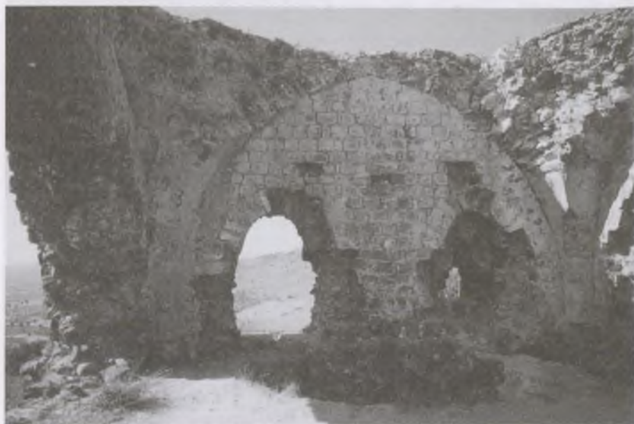
6. Burğ Zārā – interior of the first floor hall with remains of embrasures
