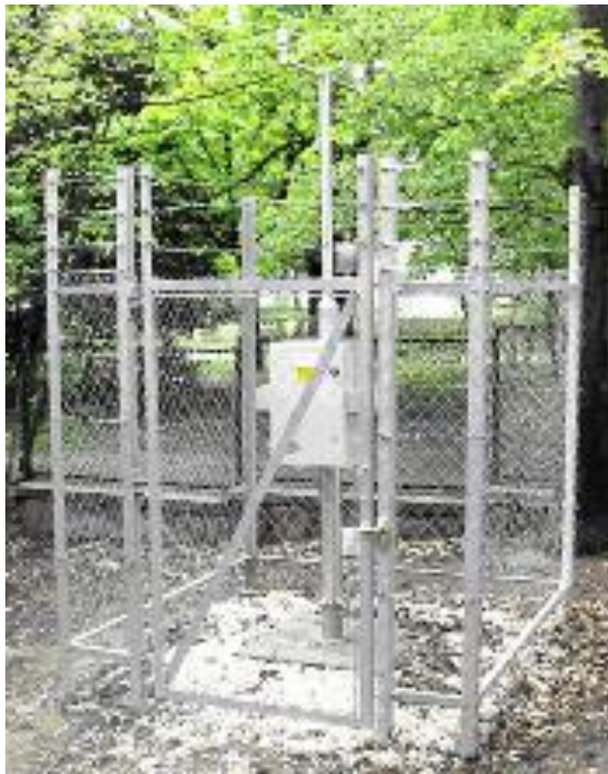
Figure 7. Deployed meteorological station with weather sensors
