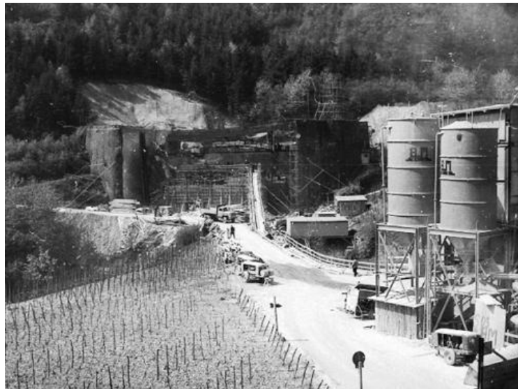
Figure 12: The construction of the largest protected command post of the Federal Republic of Germany in the 1970s [14]
