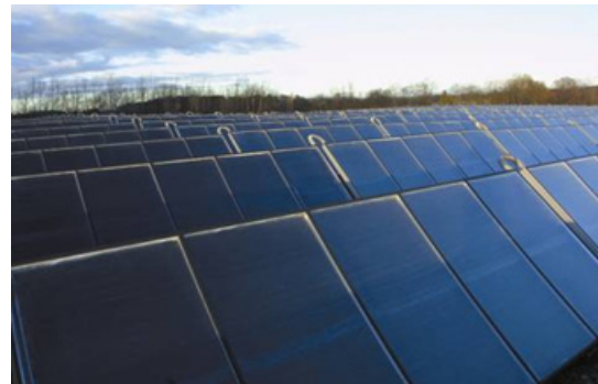
Figure 26b. Type b) Solar Thermal Collector field on the ground (Photo: ARCON/ESTIF 2016)
