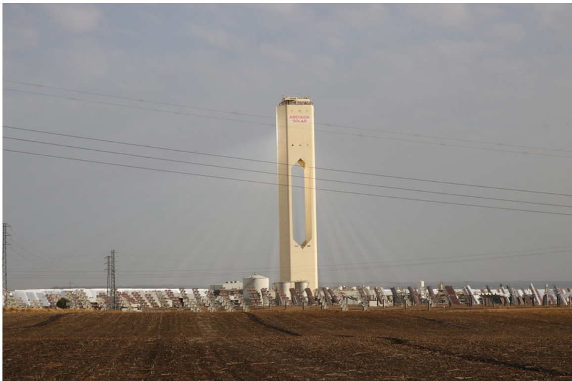
Figure 27. Solucar PS10 is the first solar thermal power plant in the world that generates electricity with this technique in a commercial way, near Seville, Spain (Photo: Naja Marot 2017)
