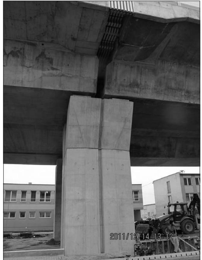
Fig. 5: Common pier 21 with expansion joint
