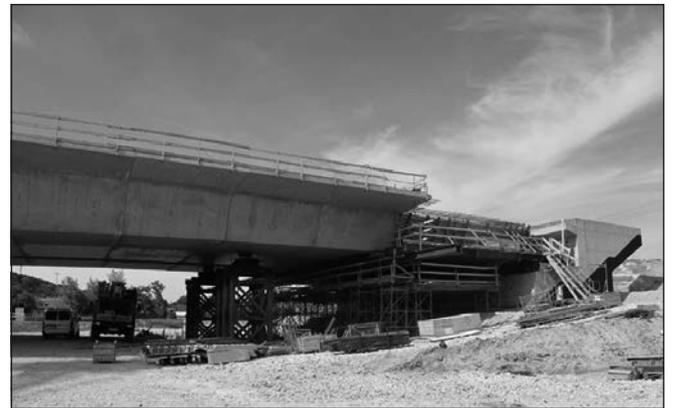
**Fig. 10:** Construction of the last segment of DC2 at abutment 26 in hanged formwork
