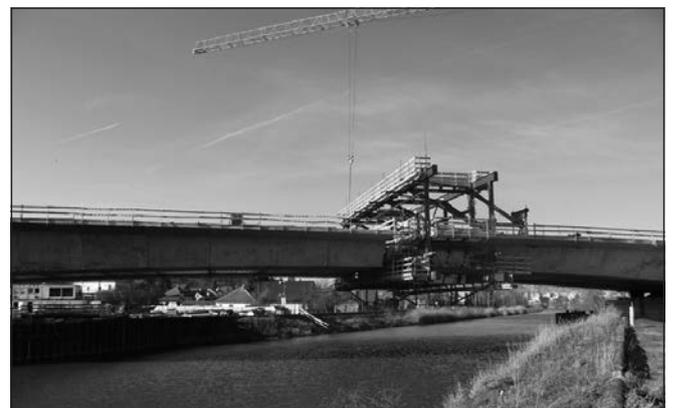
**Fig. 11:** Connection of the two arms of the DC2 bridge section above the river
