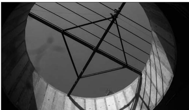
Fig. 11: Rotunda compiled with precast wall elements
