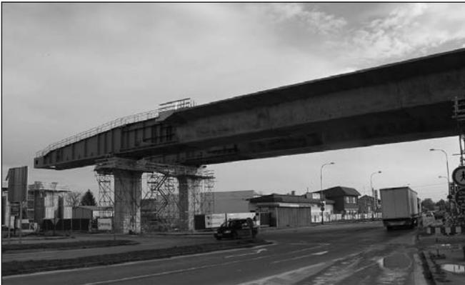
**Fig. 7:** Pushing of the DC1 bridge section above Nové Zámky road
