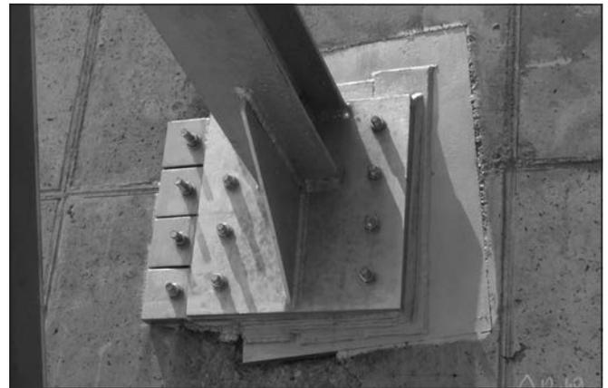
Fig. 12: Penthouse cantilever corrected joint
