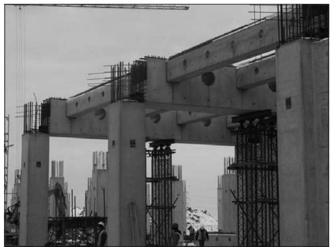
**Fig. 10:** Precast structure of the slab before concreting with temporary shoring structures
