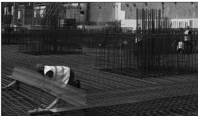
**Fig. 2:** Construction joint in the raft
