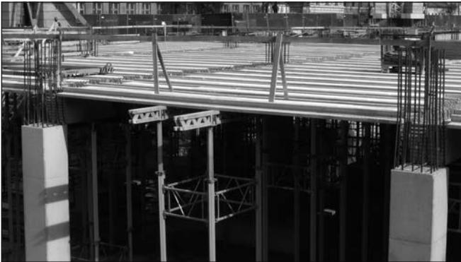
**Fig. 5:** Scaffolding of the core panels. Column-beam-slab joint before pouring
