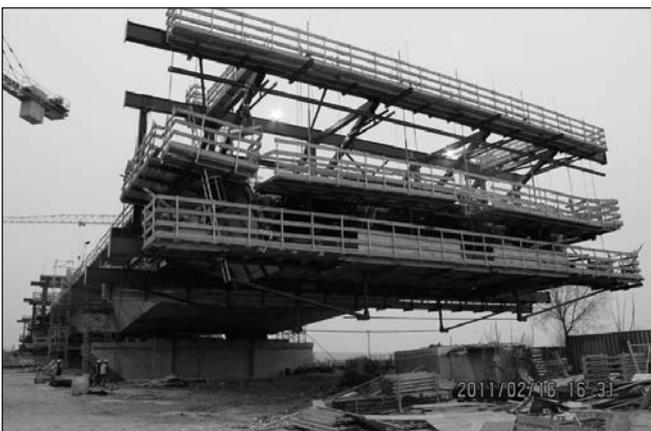
**Fig. 9:** Formwork wagon of the DC2 bridge section
