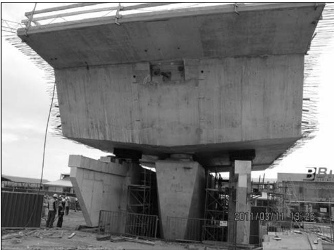
**Fig. 8:** Completed starting segment with anchor heads of transversal prestressing supported by stabilizing concrete walls
