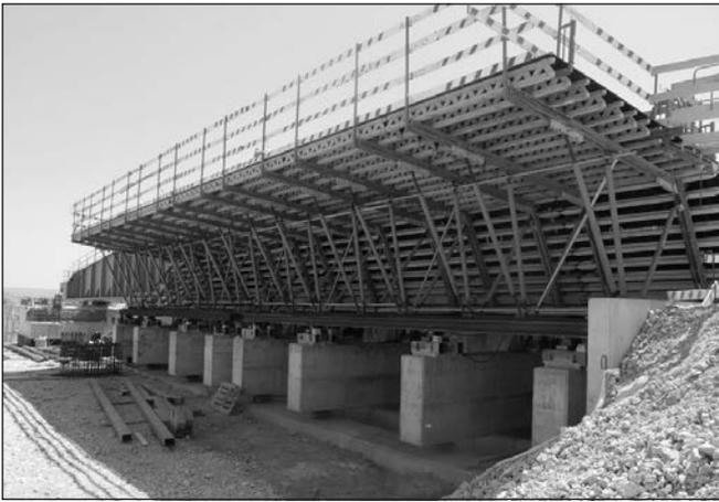
**Fig. 6:** Constructing deck of DC1 with the launching nose ready for starting
