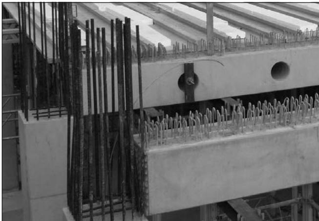
Fig. 10: Dead load reducing light fills between the ribs of the panels
