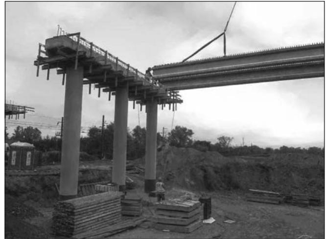
**Fig. 14:** Construction of the Komárom bypass road: lifting and positioning of the bridge girders
