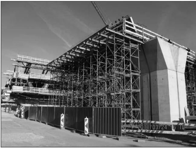
**Fig. 12:** Construction of the last segment of DC 2 at common pier 21, on heavy scaffolding
