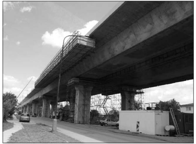
**Fig. 14:** Final works on DC1 bridge part: making of the curbs
