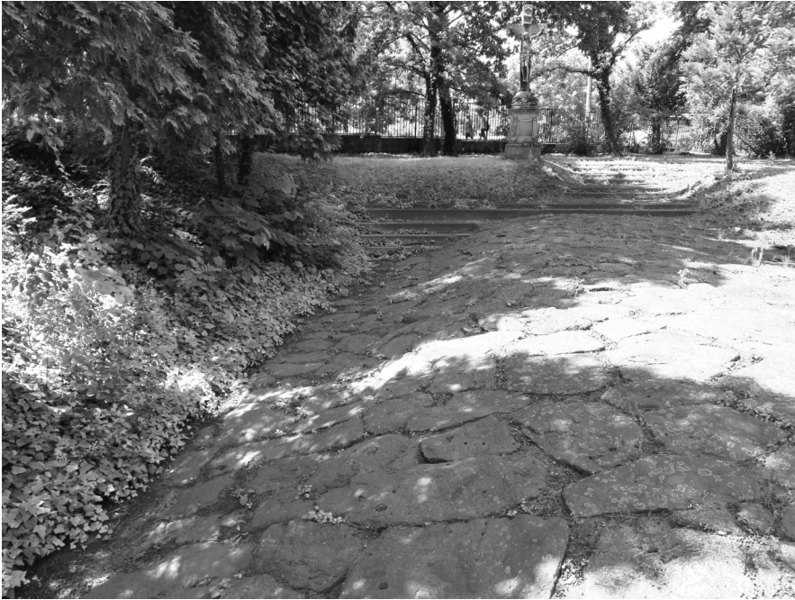
Figure 3. Uneven subsidence of a Roman road in Savaria. This kind of deformation is often caused by seismically induced liquefaction of the subsoil. Szombathely, Roman garden. #2156
