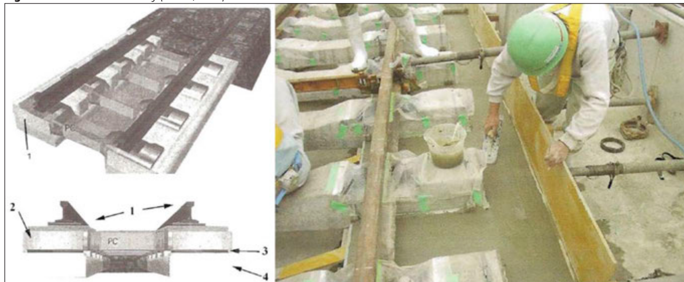
Fig 1: Elasto Ballast track railway (Ridout, 2009)
