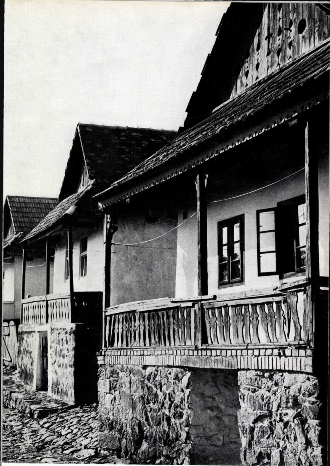
HOLLÓKŐ (Northeastern Hungary.) A uniform row of early twentieth-century houses. Steps lead down to cellars below the front porches.
