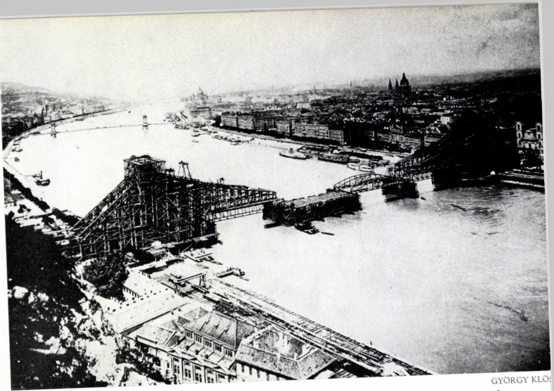
A view of Budapest with the Elizabeth Bridge under construction, taken in 1898 by György Klösz
