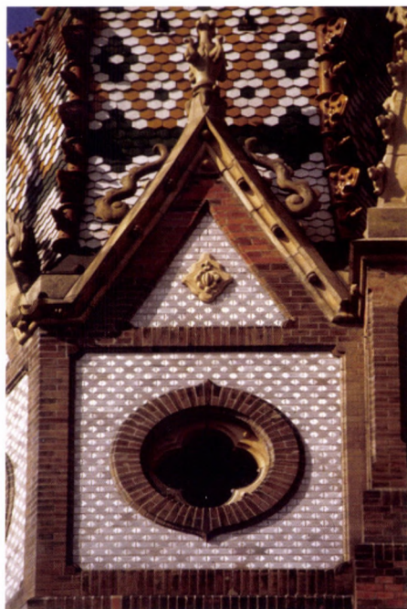
St Ladislaus Church 25 St Ladislaus Square (10 th district), Budapest Ödön Lechner, 1900
