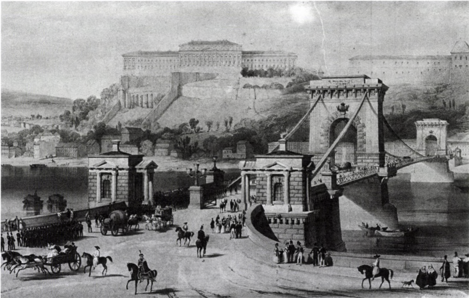
The Chain Bridge between Buda and Pest. Drawing by G. Hawkins Jr. Hungarian Architectural Museum, Budapest. From the book under review.
