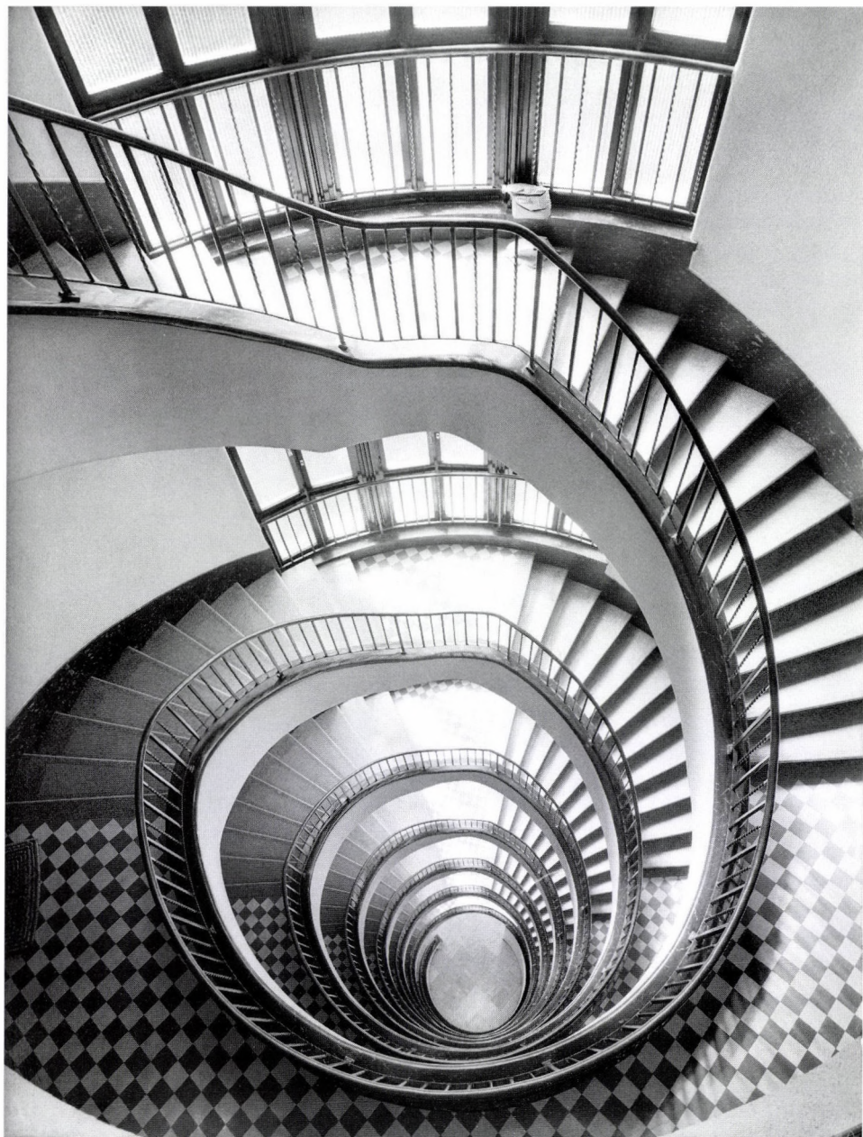
Apartment House. Pozsonyi út 53–55. Architect: István Hámor (Hamburger), 1941–1942. Vestibule. Photo: Zoltán Seidner, 1942.
