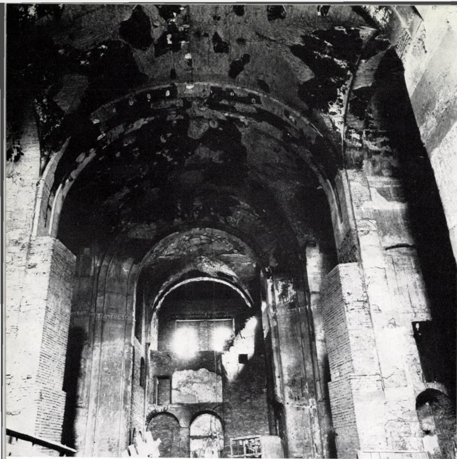
The interior of the theatre in 1968 before reconstruction was started
