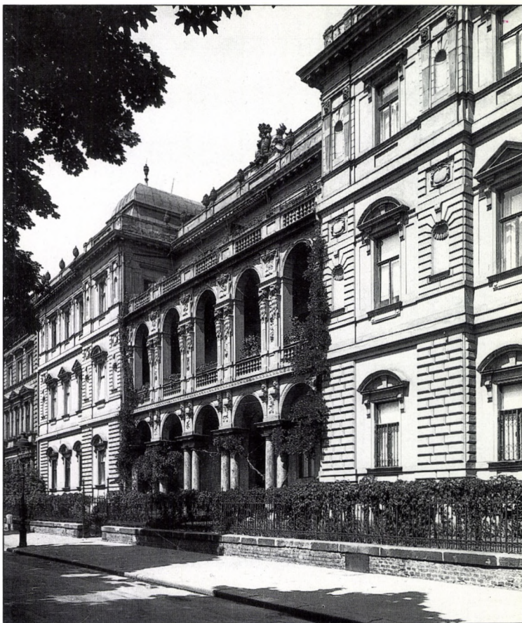
No. 98. THE PALLAVICINI HOUSE DESIGNED BY GUSZTÁV PETSCHACHER.
