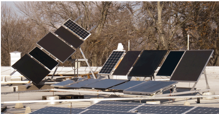
Figure 4 PV modules installed by different tilting. Fixed 12° and 42° (right) and on a 30° single axis tracker (left). Modules c-Si, a-Si, CIS, CdTe and micromorph-Si on 42° from left to right.
