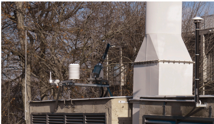
Figure 2 Integrated weather station on the roof of MEMS lab. building.
