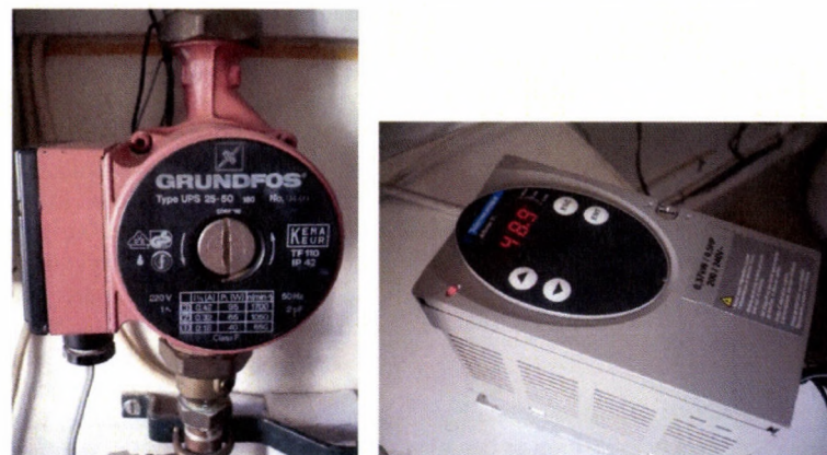
Figure 2. Pump and frequency regulator
