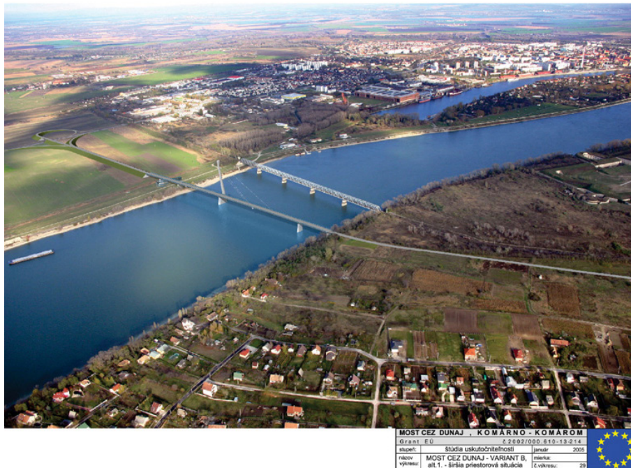
Fig.15. The planned bridge: the new axes of an evolving trans-border suburb townscape. Source: http://komarno.sk/docs/2006_04_26_interreg_29.jpg
