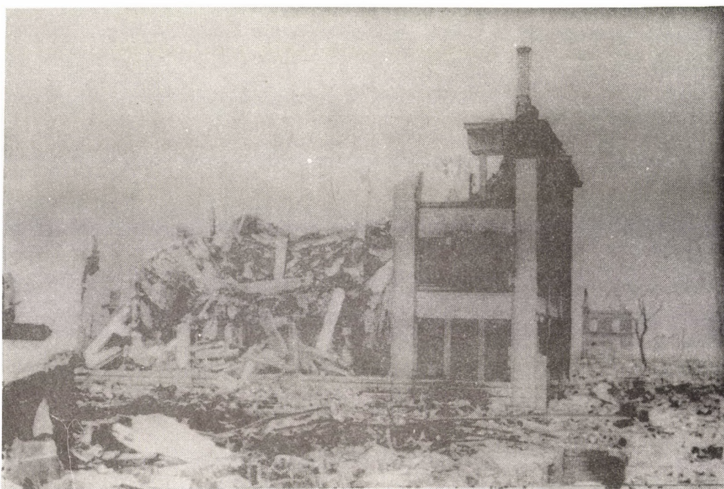
Fig. 2. Collapsed building of a bank, about 300 m southeast of the hypocenter (August 13th, 1945).
