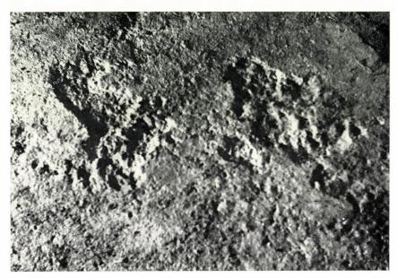
Fig. 8. Heavily worn, pitted asphalt "x" floor after use for a few months in a pig house
