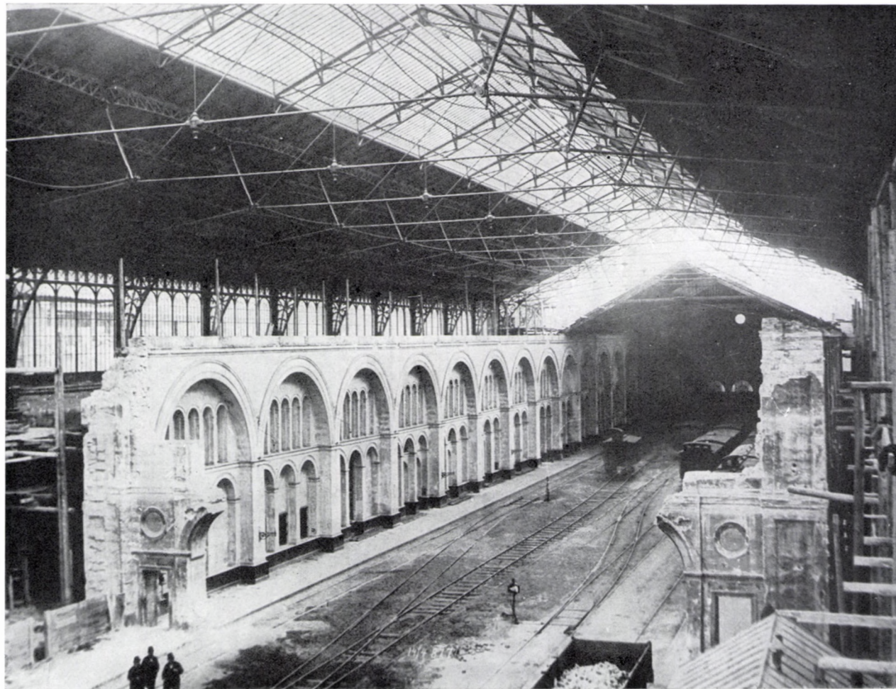
Fig. 8. Inside of the completed main hall, with the old station building while being demolished, underneath (Photo by György Klösz, 14 January 1877)
