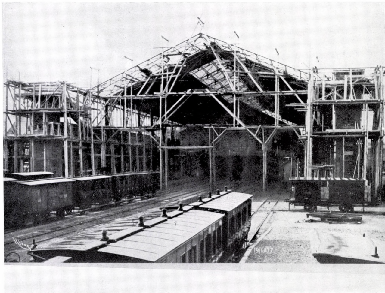
Fig. 7. Construction of the main hall as viewed from the train departure side. Underneath the old station building, in full operation all along the construction period (Photo by György KLÖSZ, 19 January 1877)
