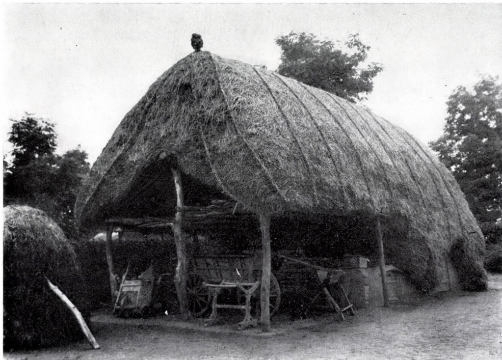
Fig. 3. Tiszaszentimre — County Szolnok — Farming outhouses: barn, summer-shed, cellars. Built in the middle of the 19th century. (Photo L. Vargha, 1936)
