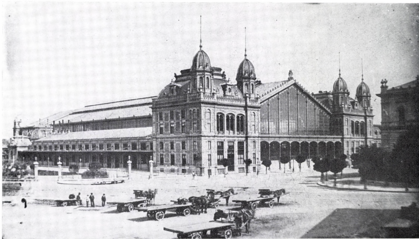
Fig. 11. Full view of the "Western Station" immediately after the completion of its building (contemporary photo)
