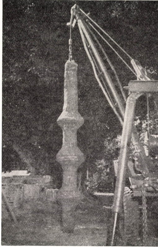
Fig. 1. Triple underreamed pile
