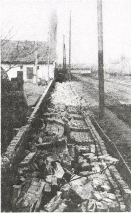
*Fig. 4.* Szigetszentmiklós, one-layer brick fence destroyed by earthquake
