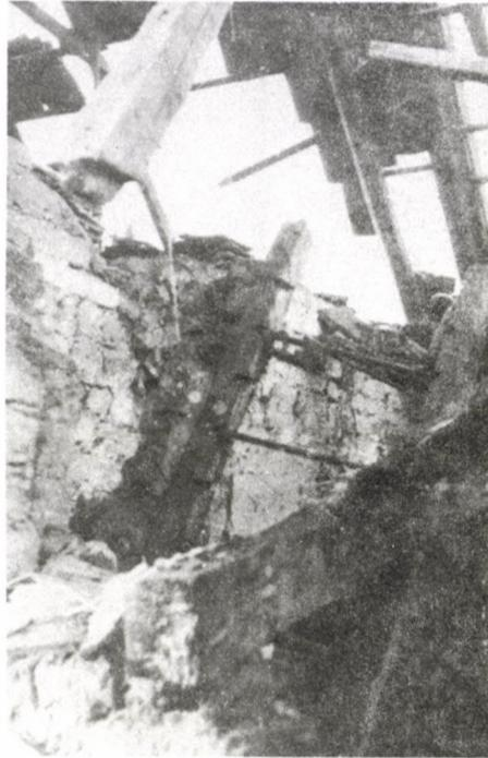
*Fig. 5.* Dunaharaszti, No. 22, Szőlőhegy Street. Destruction of a cob-wall building by the earthquake
