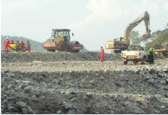
Figure 1: Dam construction project. Source: Author
