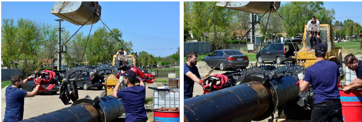
Figure 8. Installing the pipe positioning device
