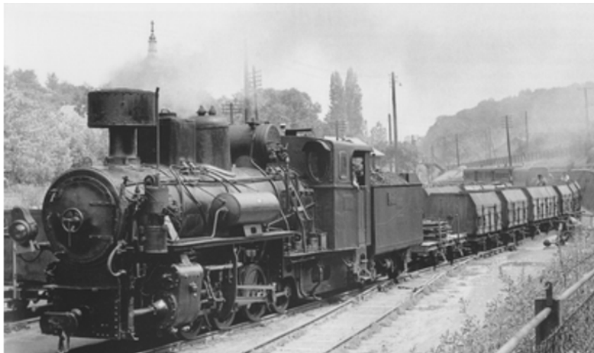
Figure 2: 1000 millimetre fitting on the line
