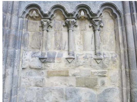
Fig. 5.: Characteristic weathering pattern, granular surface disintegration and back weathering of the Wienerwald (flysch) Sandstone on the north façade of the Ossuary in Tulln, Lower Austria (picture courtesy J. Nimmrichter).
