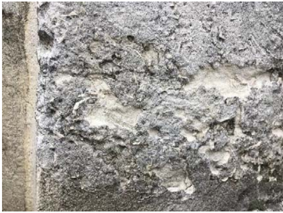
Fig. 13.: Weathering of porous biocalcarenite at the Spinnerin am Kreuz, Wiener Neustadt, Lower Austria (sample WN; picture: Pliessnig & Mozdyniewicz 2019).
