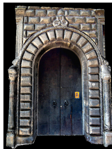
Figure 2. Palazzo Bevilacqua - Bologna three - dimensional reconstruction of a constructive detail.
