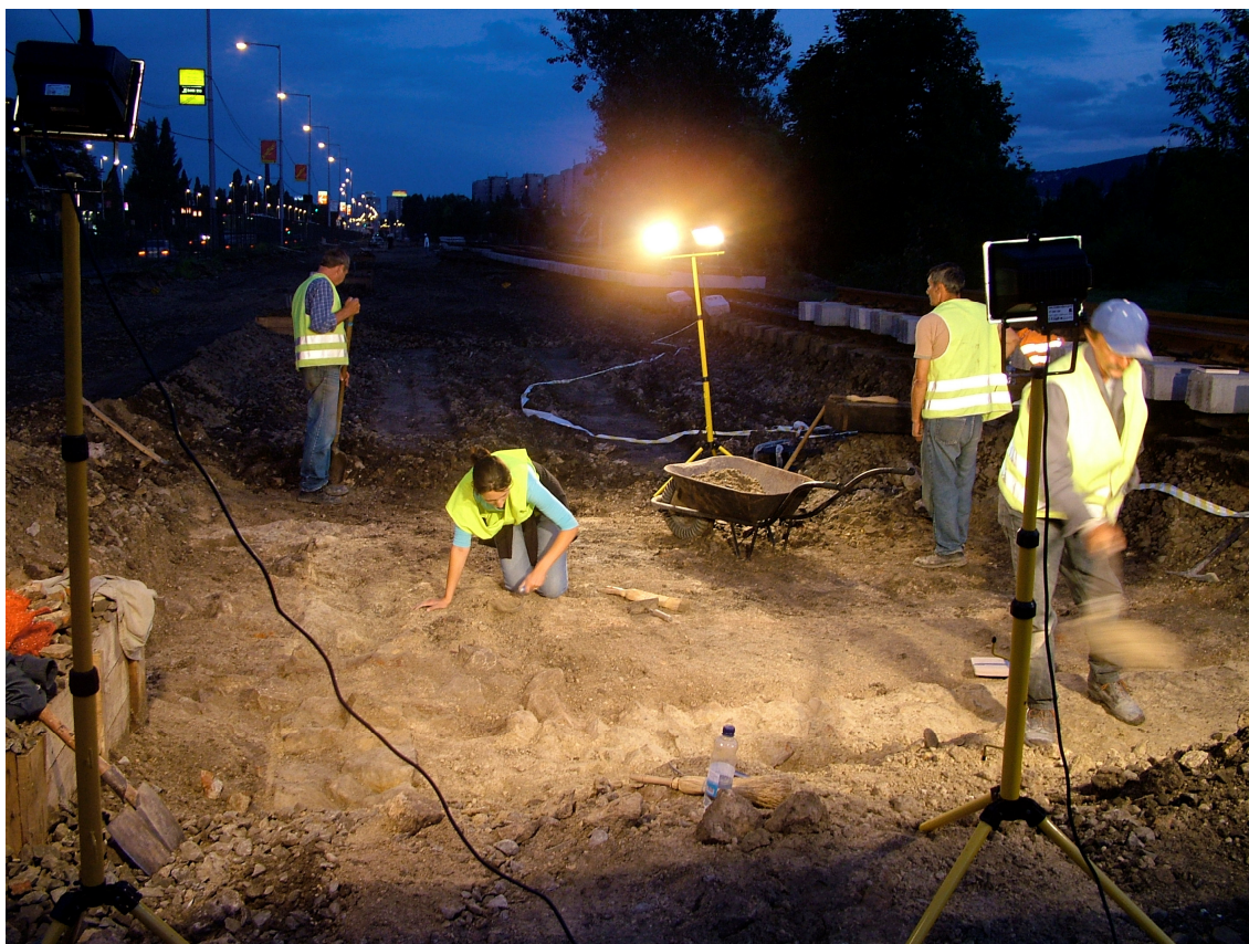
Figure 18. Excavating at night during the reconstruction of the railway line in the Civil Town of Aquincum (photo by G. Lassányi)
