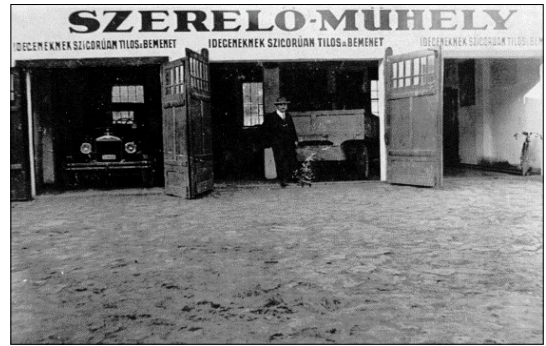
Figure 5. Ford depot from the yard in Makó.
