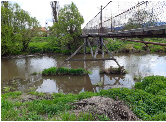
Figure 3. Pedestrian bridge on the original substructure
