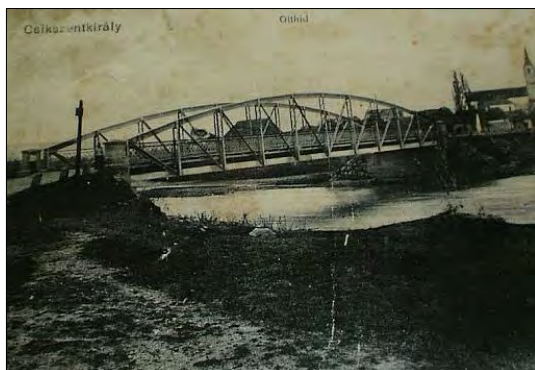
Figure 1. Postcard illustrating the former Olt bridge in Sâncrăoieni, before 1916 [1]
