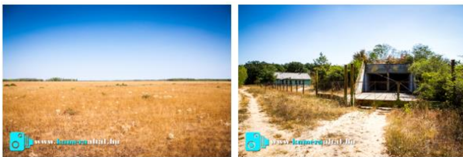
Figure 3. Kenyeri airport and the current state of the building and car cover. 14
