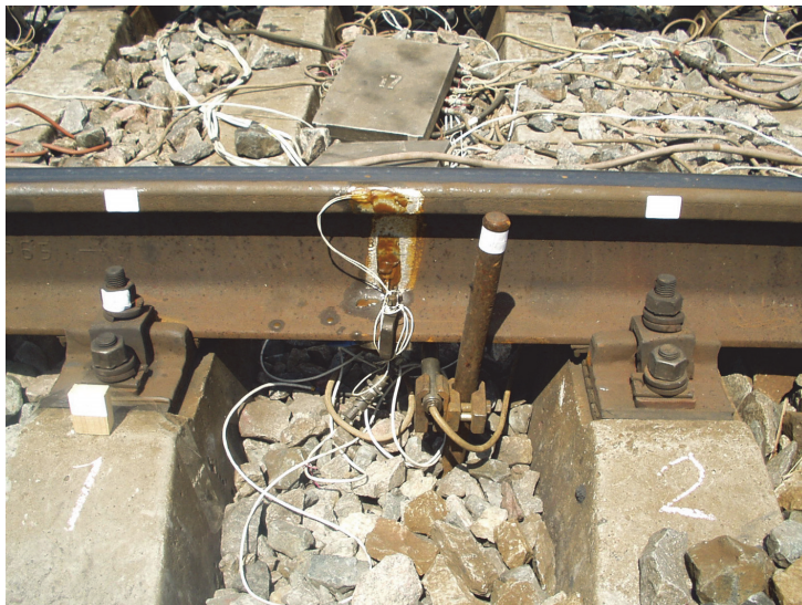
Figure 5. Installing transducers on a rail
