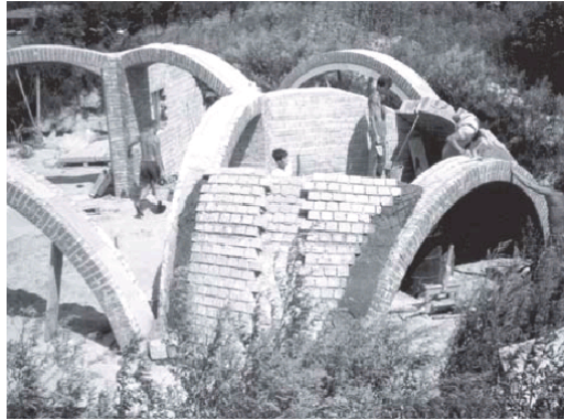
Figure 13: Masonry structure of the earth house in Tököl (Hungary) [17]
