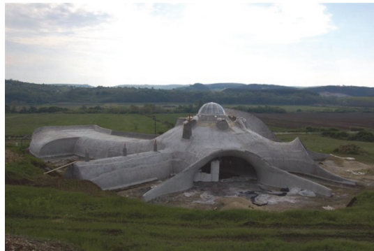
Figure 15: Supporting structure of an in-hill house (Egerszalók, Hungary) [21]
