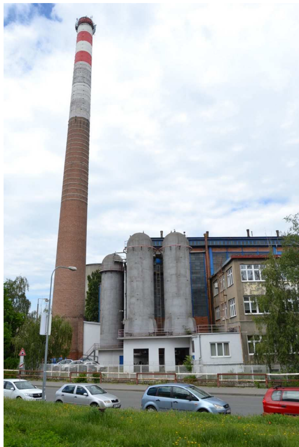
Figure 3 Area of heating plant Brno from Špitálka Street
