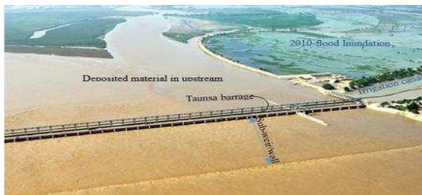
Figure 5. Aerial view of the Taunsa Barrage, construction of sub-weir, sediments in head up during the flood in 2010. (Source URL: https://www.dawn.com/news/1195398 )
