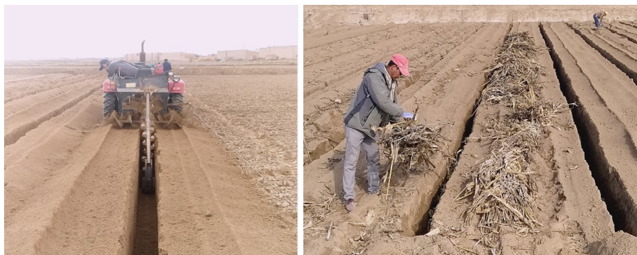
Figure 1. Blind ditch and laying cushion
