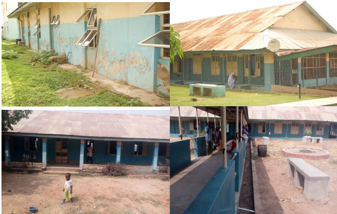
Figure 6. Exterior views of the selected wards
