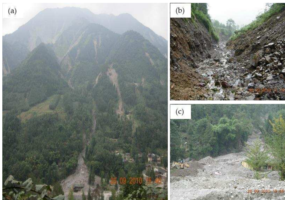
Figure 3. (a) Photography showing the whole Shuida catchment and co-seismic landslides developed upslope; (b) The debris-flow scoured channel; (c) The deposited fan
