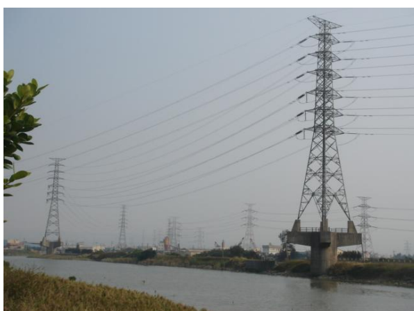
Figure 26. No. 10 and No. 12 towers
