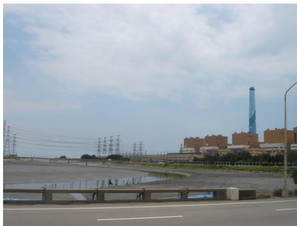
Figure 2. Tower cables to external connections
