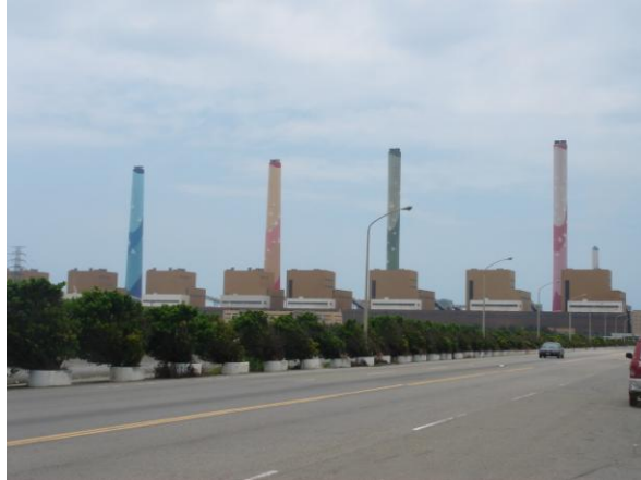
Figure 1. Taichung Power Plant
