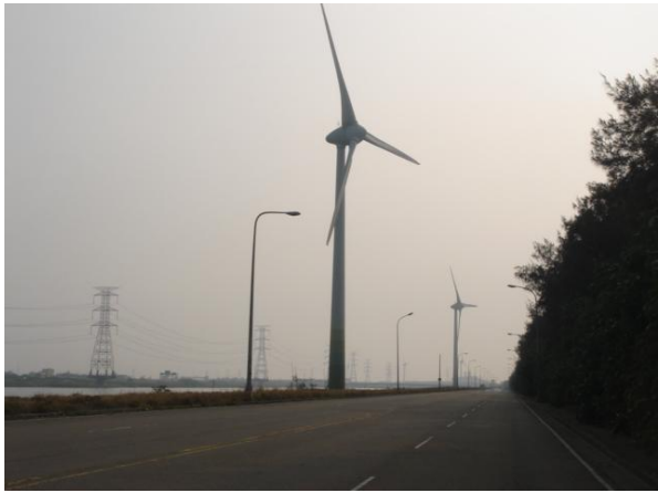
Figure 16. No. 34 wind turbine
