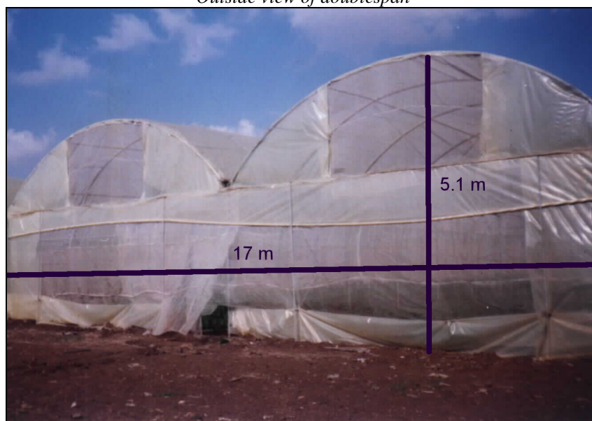
Outside view of doublespan
