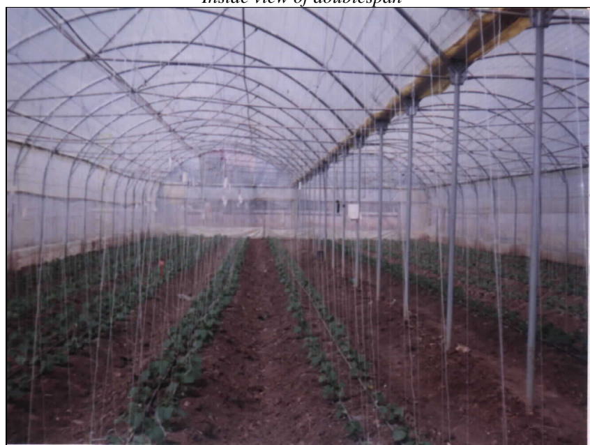
Figure 2. Doublespan plastic house having two round-arches (5.1 m height, 17 m width and 55 m length) covered an area of 935 m 2 .
