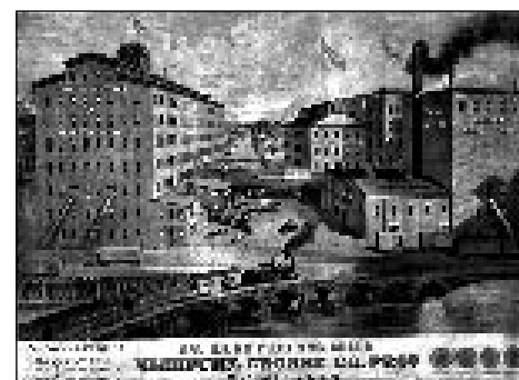
Washburn A malom, Minneapolis, 1880. Mill Washburn A, Minneapolis, 1880.
