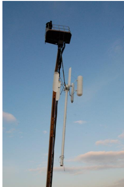
Figure 9. Craning of Vertical Axe Wind Turbine (VAWT) at Óbuda University
