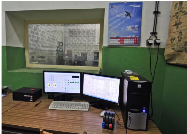
Figure 2 The control room and control computer
