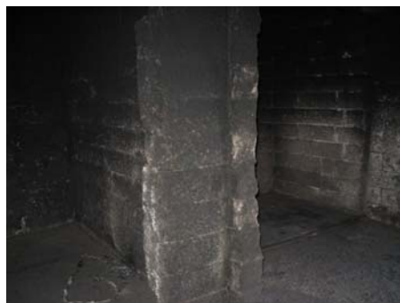
Figure 3 Measurement room interior
