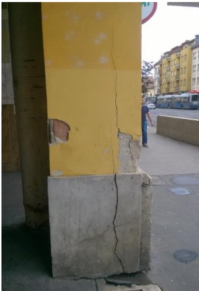
Figure 1: Vertical crack in the masonry pier of a multi-storey building (Made by: Péter Tóth)
