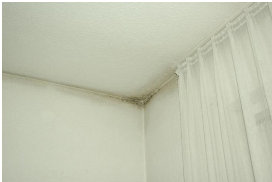
Figure 10: Mold due to cold bridge wall structure (Made by: Péter Tóth)
