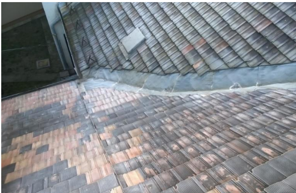
Figure 6: Worn out zinc sheet valley (Made by: Péter Tóth)
