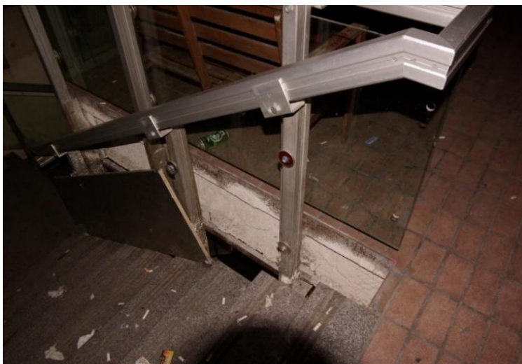
Figure 12: Incomplete, poorly maintained handrail in a nightclub (Made by: Péter Tóth)
