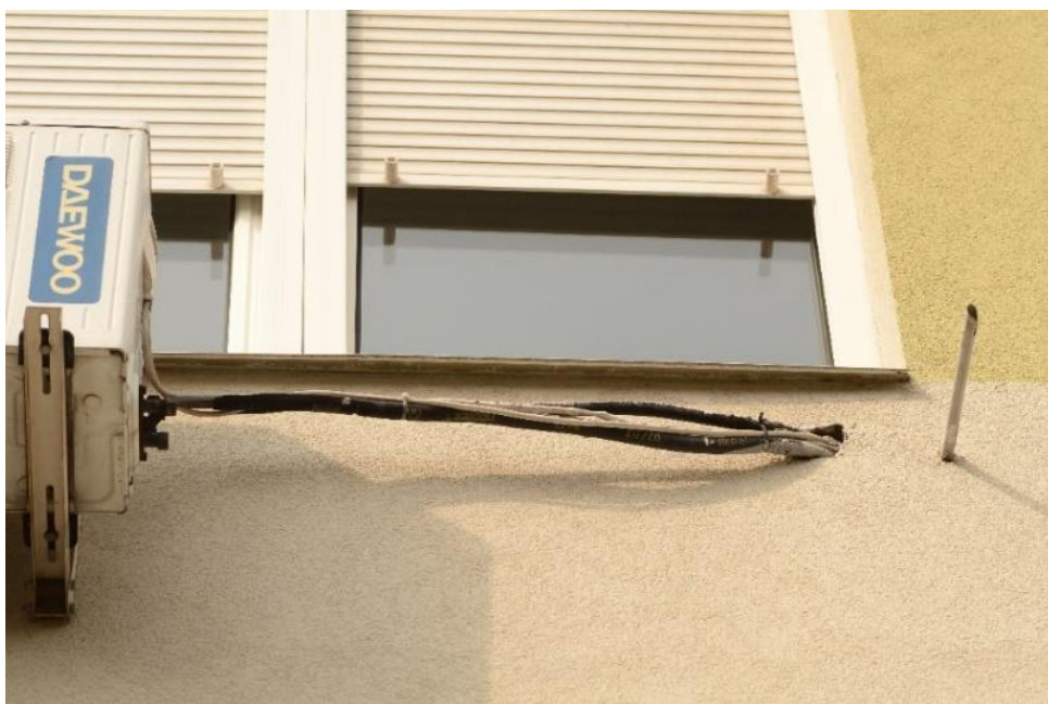
Figure 7: Due to the installation of air conditioning equipment, the façade thermal insulation system was broken through, and the seal was solved with PUR foam. (Made by: Péter Tóth)
