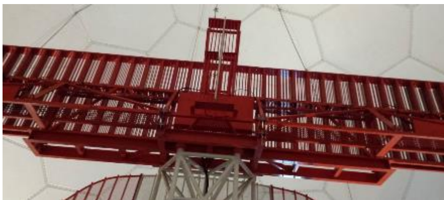
Fig.16 MSSR LVA Antenna Back Radiator [9]
