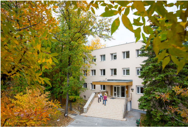
Figure 1: Central building of the EK
