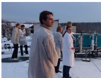
Figure 1: Training on ICP-MS, air-handling system on the roof of building 17/A
