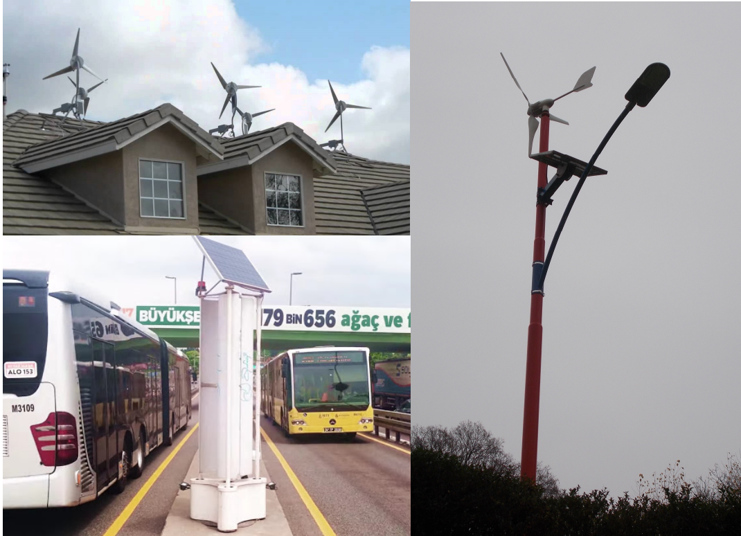
Figure 5. Wind turbines in urban regions: a, Roof-mounted WTs [9]; b, Mini wind turbine and solar cell on a street light pole in Budapest [10]; c, VAWT and solar panel between passing vehicles in Istanbul [11]
